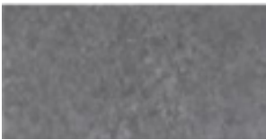
BS2020/19201 Rugged Concrete
